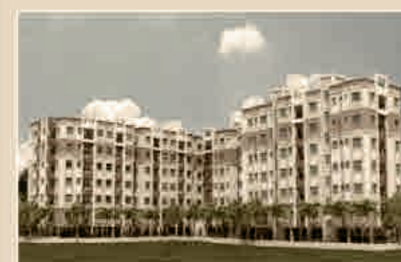
GREEN OASIS - KAIKHALI, KOLKATA
