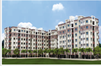
GREEN OASIS - KAIKHALI, KOLKATA
