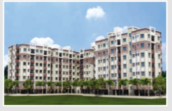
GREEN OASIS - KAIKHALI, KOLKATA
